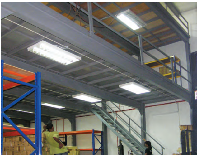
Multi-tier Steel Platform System
